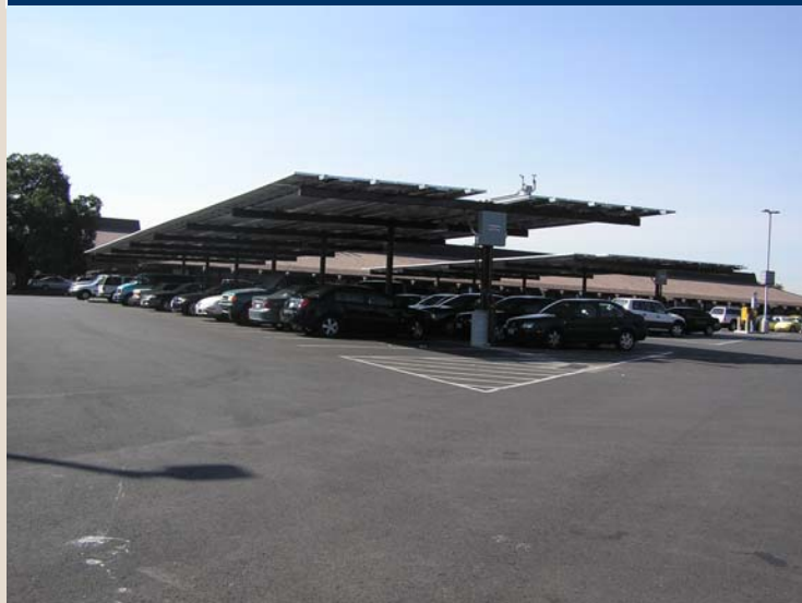
PV Shade Structure
